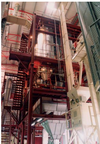
Continuous Parboiling Plants in Greece (Large and small capacity)
